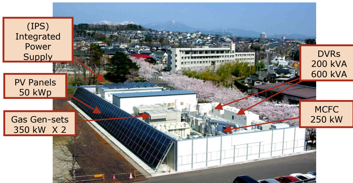
Overview of Sendai Microgrid
